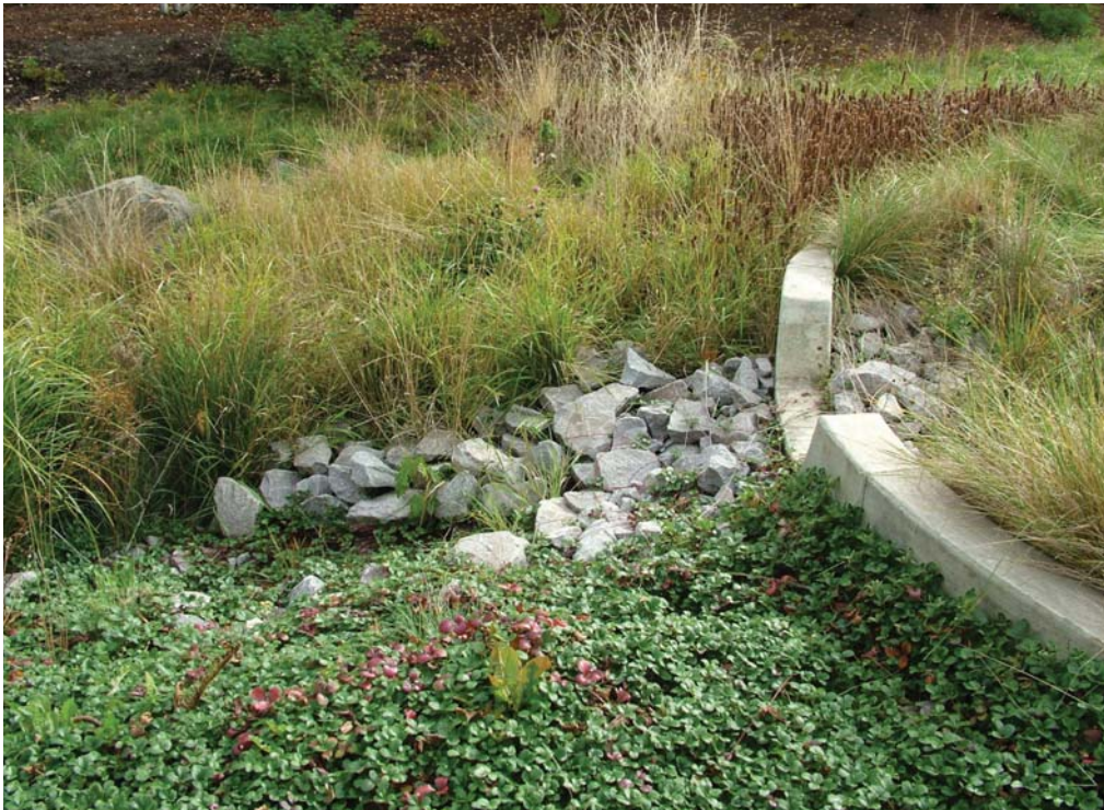
Ornamental grasses and other plantings protect this City of Portland vegetated swale from washouts.
